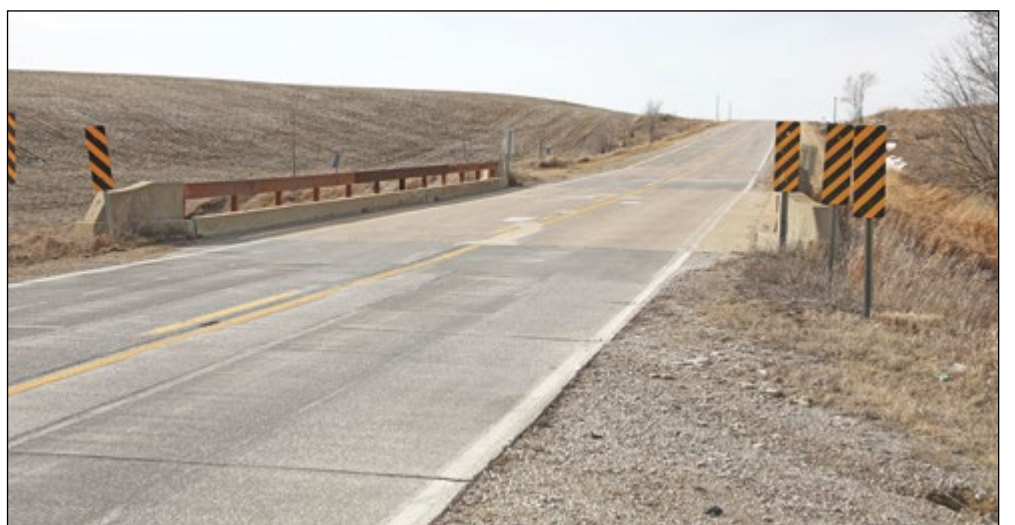
This bridge on County Road E16 will be replaced during the coming construction season.
