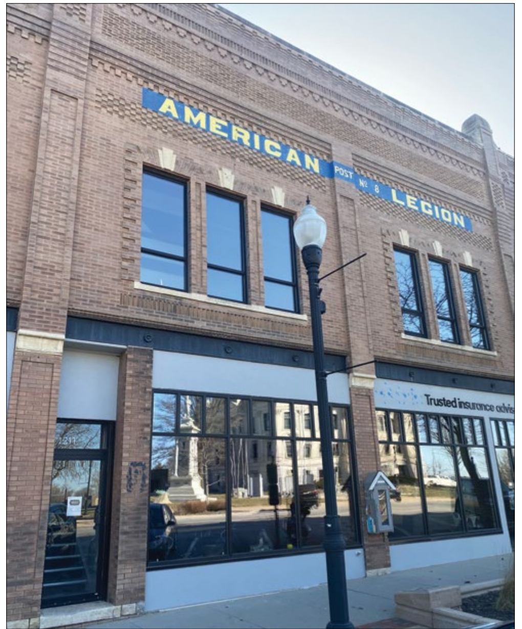
The exterior of a developing complex that will include The Old Fashioned bar and a relocated Crawford County Abstract.
