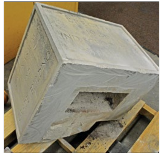
The left side of the cornerstone says, "Gymnasium and Grade Building." The hole in the bottom is where the time capsule was located. The side of the capsule at the opening to the hole had rusted.
