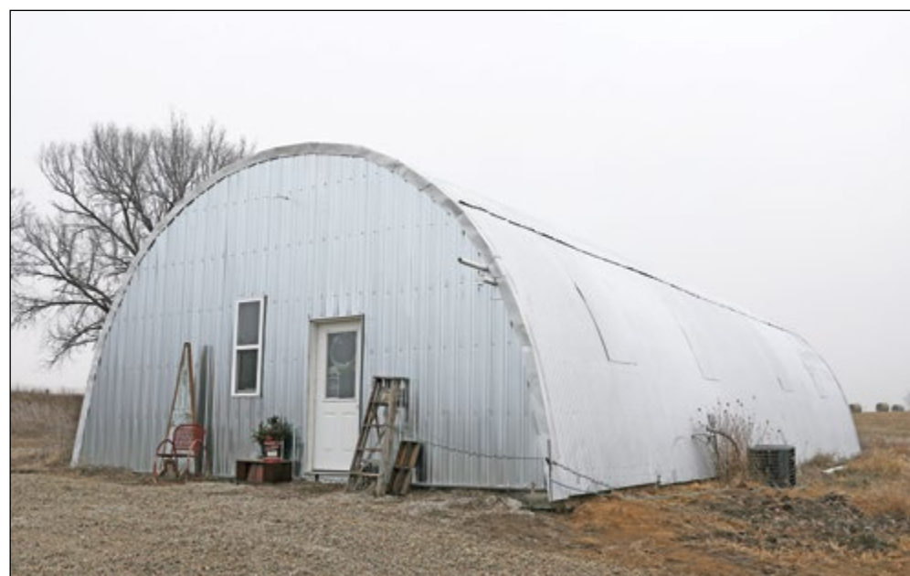
Rural Road Trading Co. and a workshop are located in the Quonset hut.
