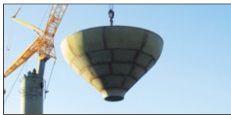
Water tower constructed
