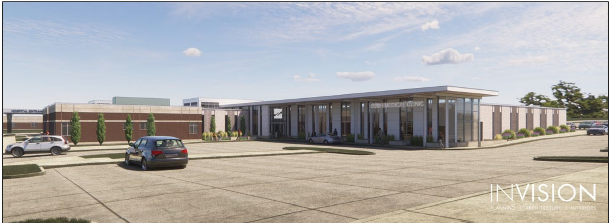
The new clinic entrance area will feature a large overhang above the walkway to protect patients from the weather. The walkway will run parallel to the clinic waiting room.
